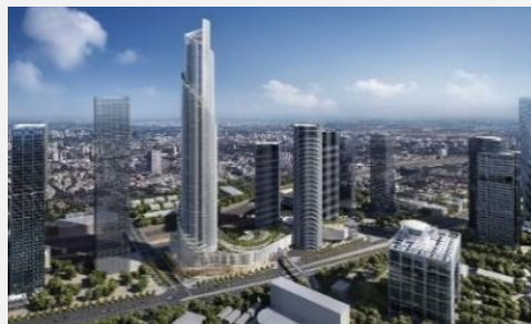
Tel Aviv Expansion of Azrieli Center and Spiral Tower ~150,000 sqm (3)
